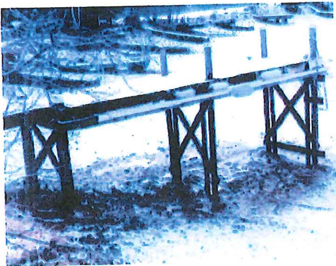
Dock Seventeen Repaired
