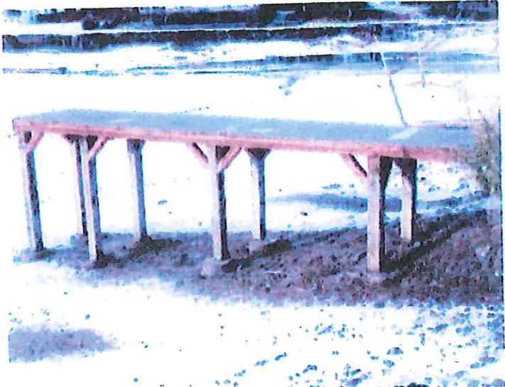
Dock Twenty Repaired
