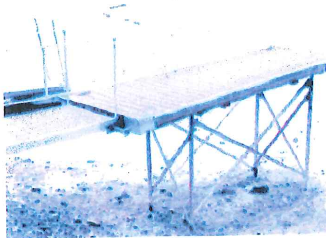
Dock Twenty-three Repaired
