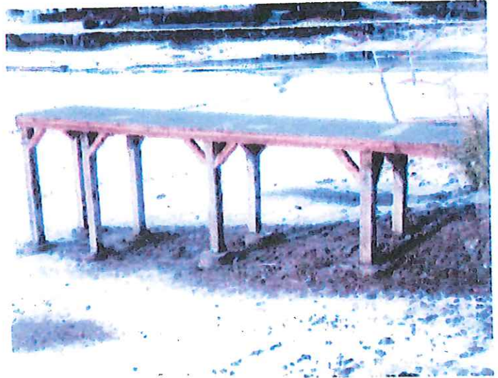
Dock Twenty Repaired
