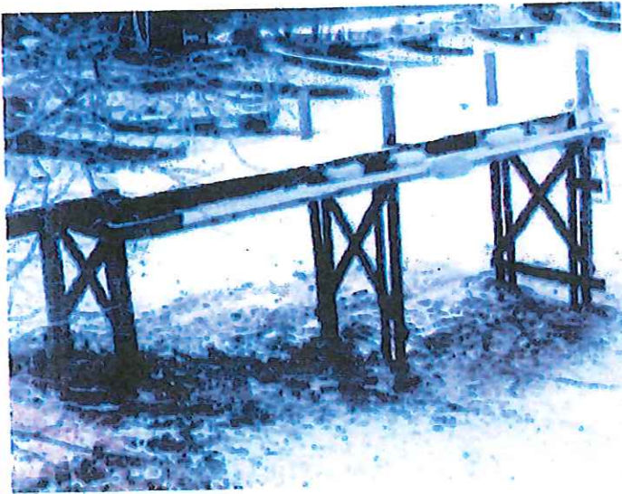
Dock Seventeen Repaired
