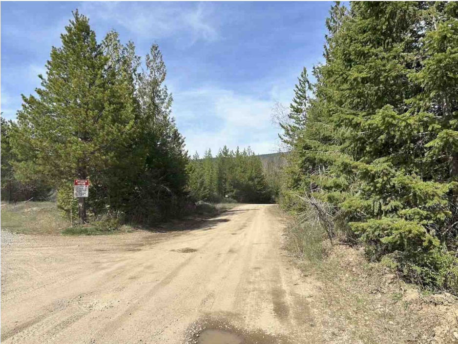
Access road past Sundance Ldg
