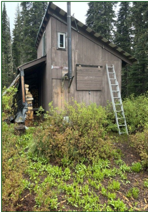
Existing structure as of June 2026
