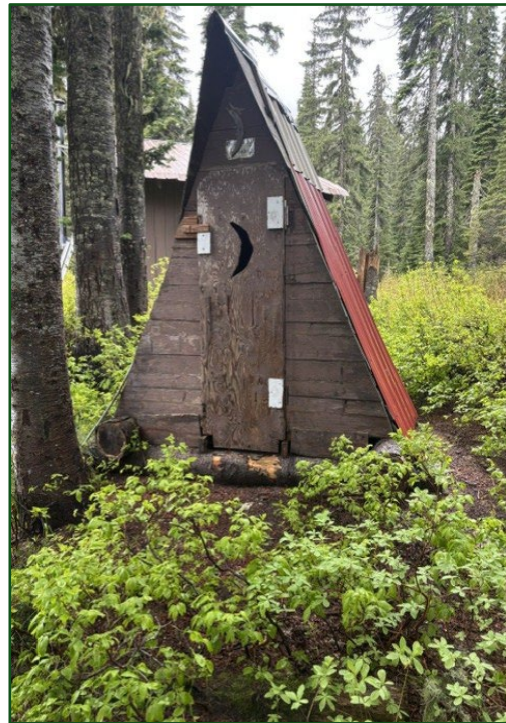
Existing structure as of June 2026
