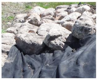
4. The riprap and filter layer must be **keyed** into the bed below the high water mark.
