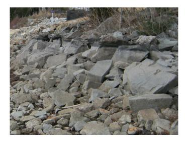
2. Riprap shall be placed along the **present contour** of the shoreline; however, riprap shall not be placed on a slope steeper than 1.5H:1V.
