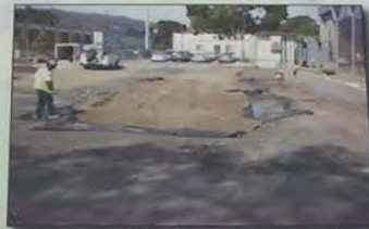
The rain garden uses a special soil mixture that helps runoff soak into the ground and plants that do well in wet conditions.
