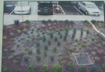
During very heavy storms, runoff ponds up and eventually overflows into the storm drain inlet to prevent flooding.
