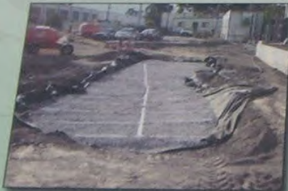
The underdrain system beneath the rain garden carries treated stormwater runoff to Brisbane Lagoon and out to the Bay.
