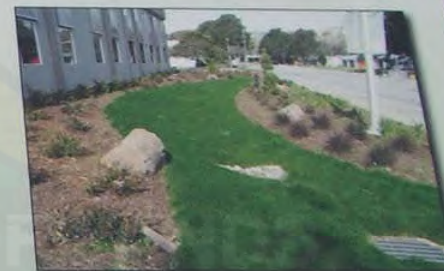
The bioswale along Valley Drive also collects and treats stormwater runoff.
