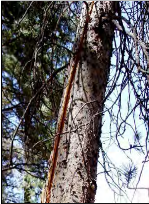
Figure 75. Recent trunk crack after high wind. The crack is deep, and the lengthwise split and some cross-grain splintering at the recent bend indicate structural failure (FP4).
