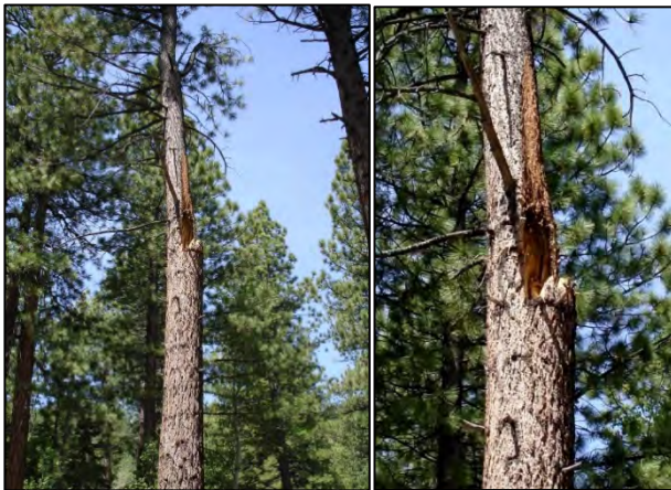
Figure 79. The remaining stem of the failed “V-fork” in Fig. 78. Failure potential of the surviving top remains high from decay, outward bend, and flattened cross-section where the failure occurred.
