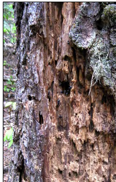
Figure 88. Carpenter ants in decayed wood.
