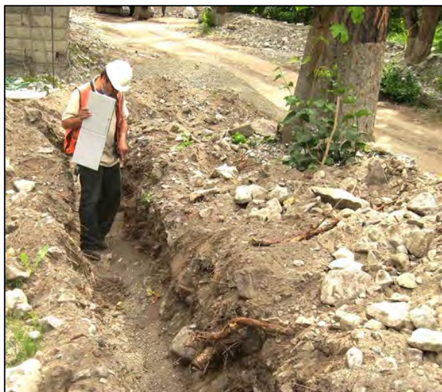
Figure 32. Excavation to install a utility line severed many of this tree's roots. Compaction and burying the base of the tree (see soil line on trunks) may have further weakened the root system.
