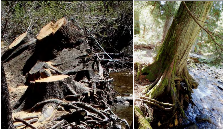
Figure 31. Undermined root systems: At left, trees were felled because of undermining and failure. Failures were away from the undermined side. At right, undermined roots of a western redcedar show ice damage common to trees along streams with winter freezing.
