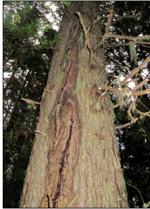
Figure 76. Western redcedar with cracks, cause unknown.
