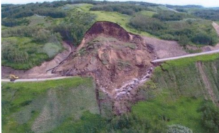
Figure 10. Deep-seated landslide showing the head scarp, body, and toe. Cecil Lake, British Columbia.
