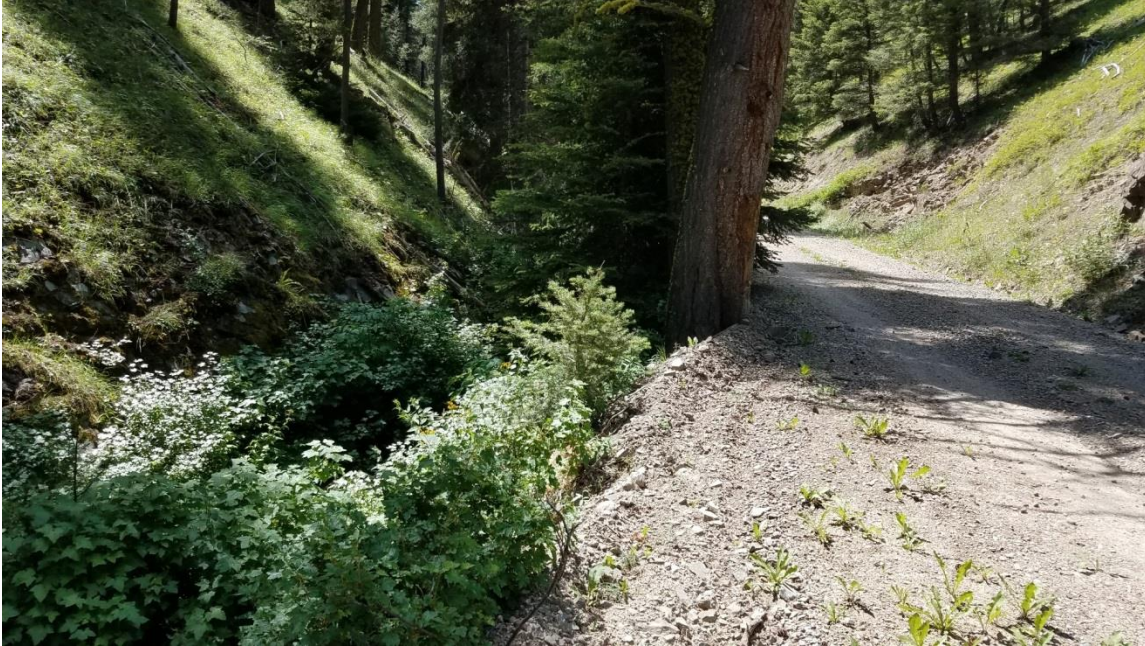
Figure 17 Long berm of grader debris being pushed into the stream
