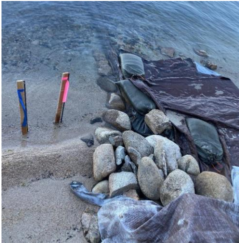
Picture 2: Taken on 7/1/22. The Wilsons barrier/jetty made of rocks, sand bags, logs and tarp persisted lakeward of the high water mark (stake with blue flag).
