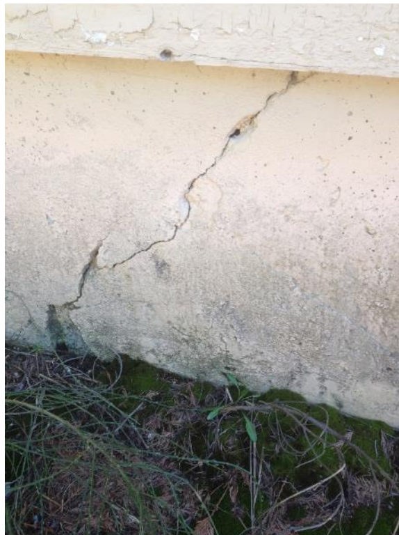
Photo 12. Building 4 – Garage. Crack in foundation.
