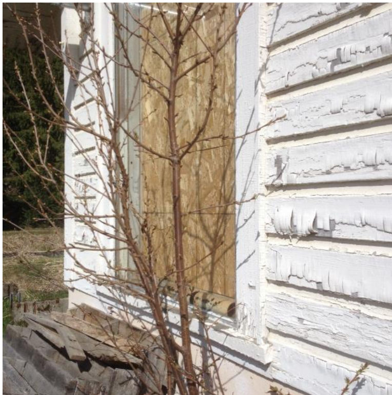
Photo 6. Building 2 – Hatchery Exterior. Peeling Paint.
