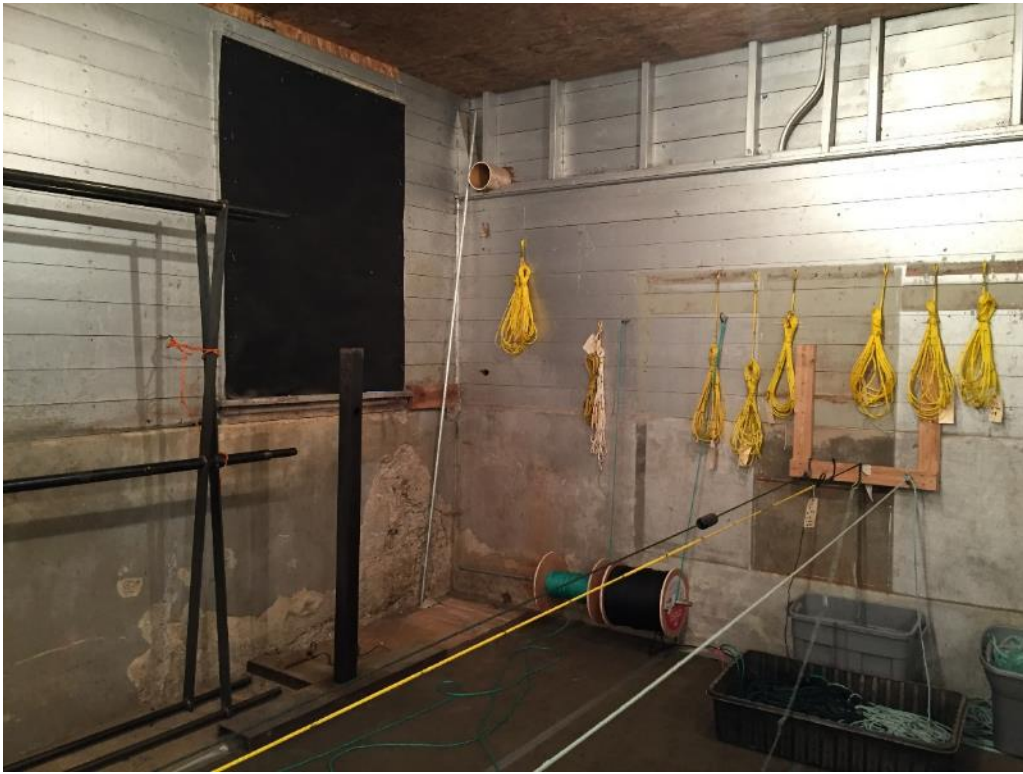
Photo 5. Building 2 – Hatchery Interior. Concrete spalling.
