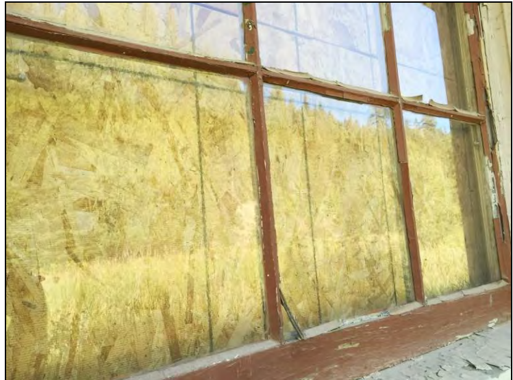
10. View of the asbestos-containing window glazing found on the exterior windows of the Hatchery Building. Also show the reddish-brown trim paint that contains lead levels above the EPA/HUD guideline regulatory limit.
