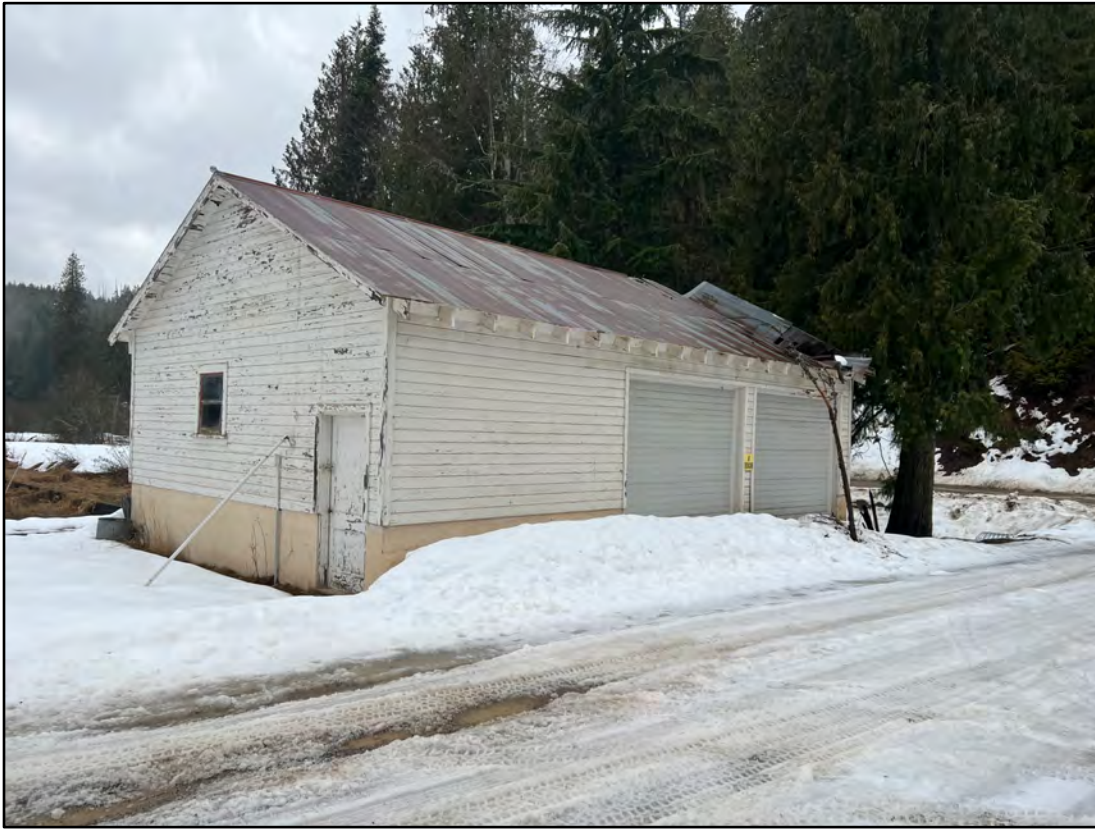
Photo Date: January 17, 2023 By: HSC View of the West Garage. Raceways apparent at left edge of frame. Spring Creek Road visible at right edge. The roof has a significant void from prior tree fall.
