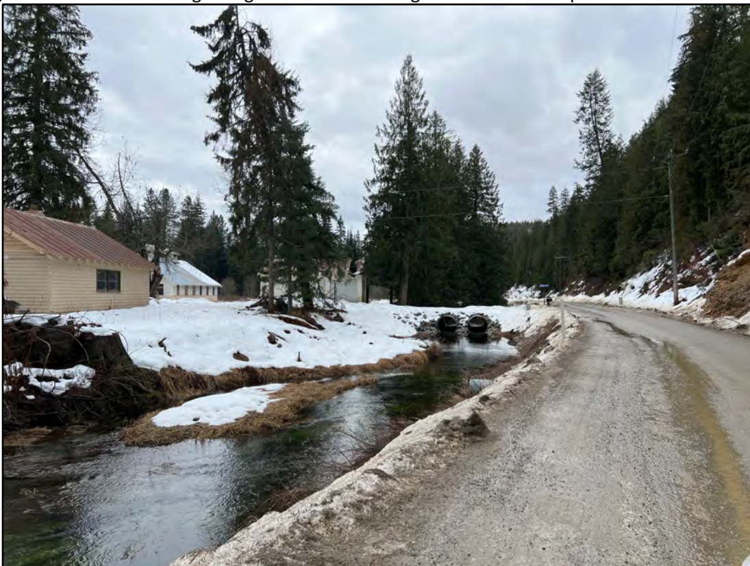
Photo Date: January 17, 2023 By: HSC View from the north looking south along Spring Creek Road. The culverts were placed following a washout in the spring of 2017.
