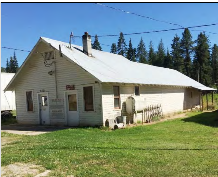
29. View of the Shop/Freezer Building showing the off-white paint that was found on the exterior siding and trim found to contain lead levels above the EPA/HUD guideline regulatory limit.
