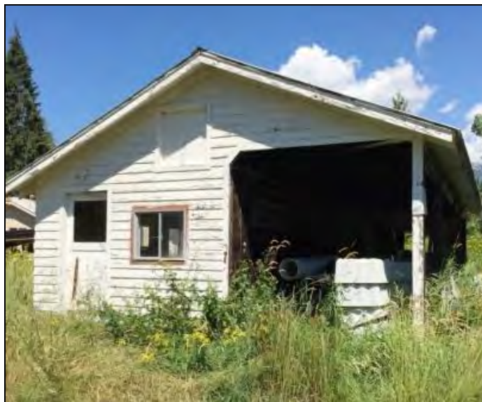
32. View of the peeling and flaking exterior lead-containing paint found the rear of the Summer Quarters.
