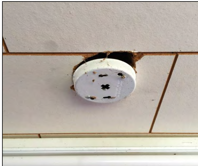
34. View of the 12-inch by 20-inch ceiling tiles found within the Summer Quarters.
