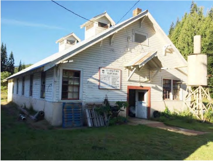
9. View of the Hatchery Building showing the off-white paint that contains lead levels above the EPA/HUD guideline regulatory limit. Also shows the non-asbestos stucco finish applied to the concrete foundation walls.
