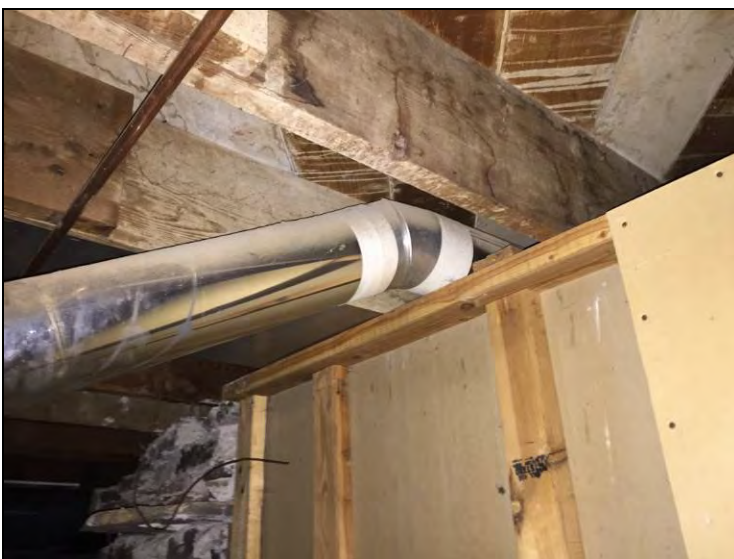
17. View of the asbestos paper duct tape applied to the exterior of the metal heat ducts found within the basement and crawlspace areas located within the Main House.
