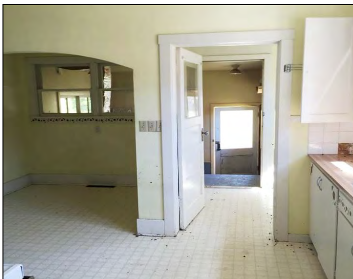
20. Interior of the Main House kitchen, dining and laundry areas located on the main level, showing the newer non-asbestos sheet vinyl flooring and non-ACM ceramic tile grout.
