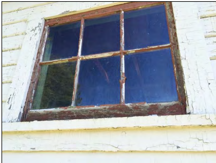
28. View of the West Garage showing the non-asbestos window glazing compound used on the exterior windows.
