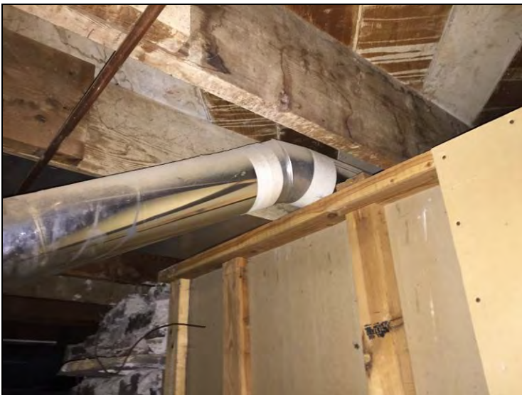
17. View of the asbestos paper duct tape applied to the exterior of the metal heat ducts found within the basement and crawlspace areas located within the Main House.
