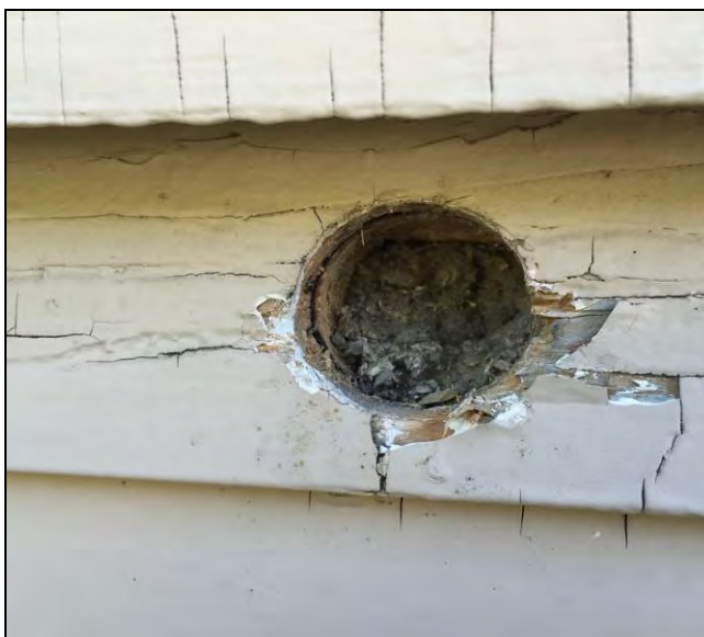
18. View of the non-asbestos blown-in insulation found within the exterior walls of the Main House. This material is similar in appearance and texture to that found within the attic space.
