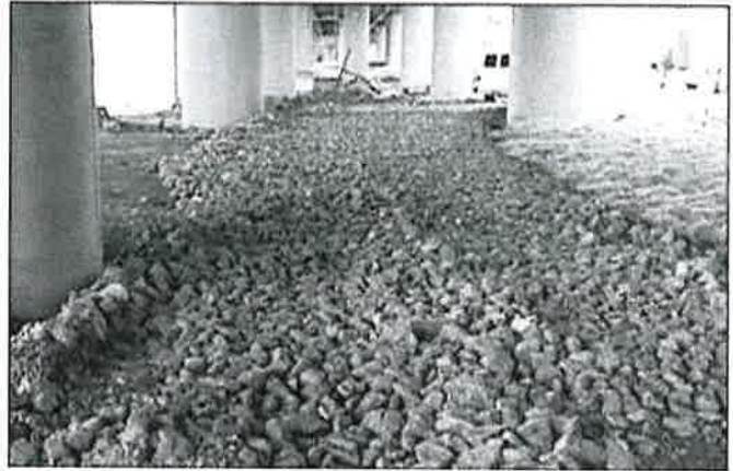
Figure 108. Temporary construction access road (ITD 2014).
