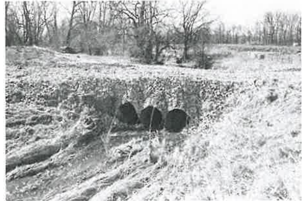
Figure 149. Temporary stream crossing using culverts (Ohio EPA 2014).
