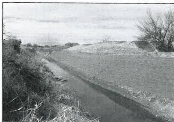
Figure 123. Geotextile channel lining (ITD 2014).
