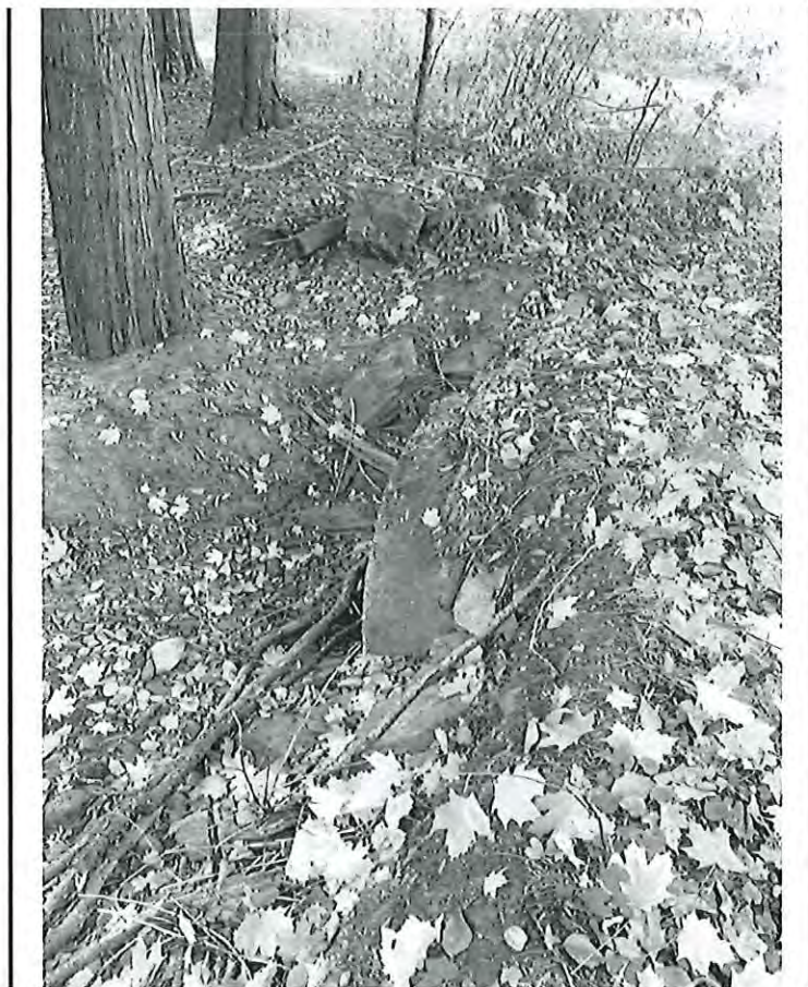
#1. North Branch inlet culvert
