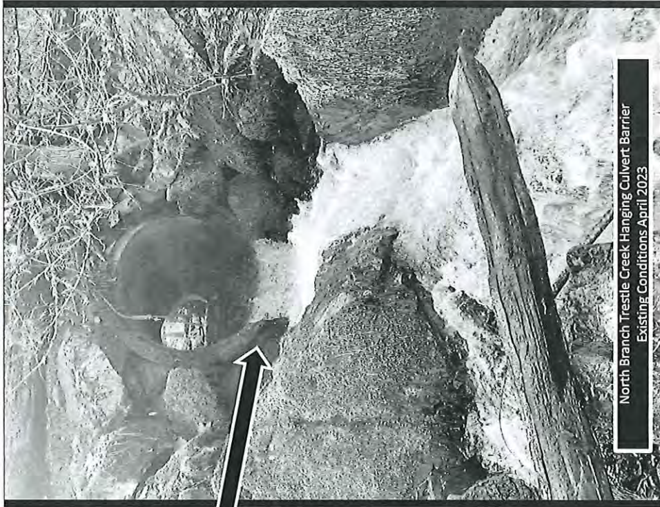
NBTC Hanging Culvert Existing Conditions April 2023
