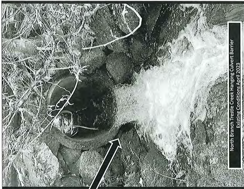
NBTC Hanging Culvert Existing Conditions April 2023
