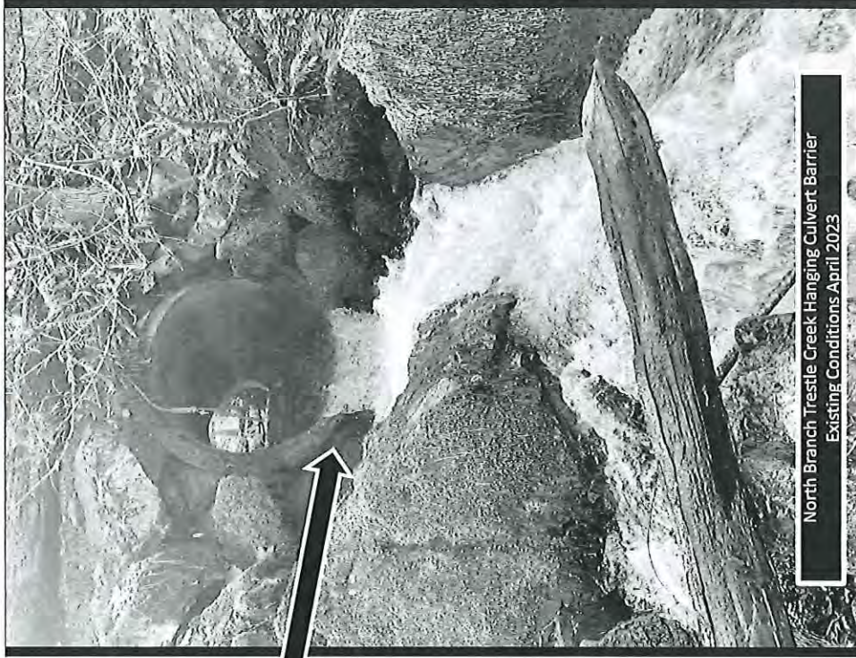
NBTC Hanging Culvert Existing Conditions April 2023
