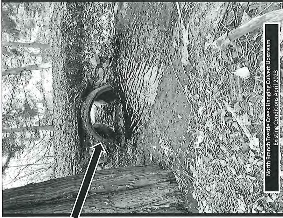
NBTC Hanging Culvert Inflow Existing Conditions April 2023
