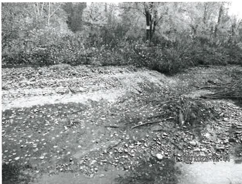
Photo 2: Looking North across slough to “Island”. Fill material consists of silts, sands, and cobbles. Water in slough drainage is rain water runoff flowing towards lake water to the left.
