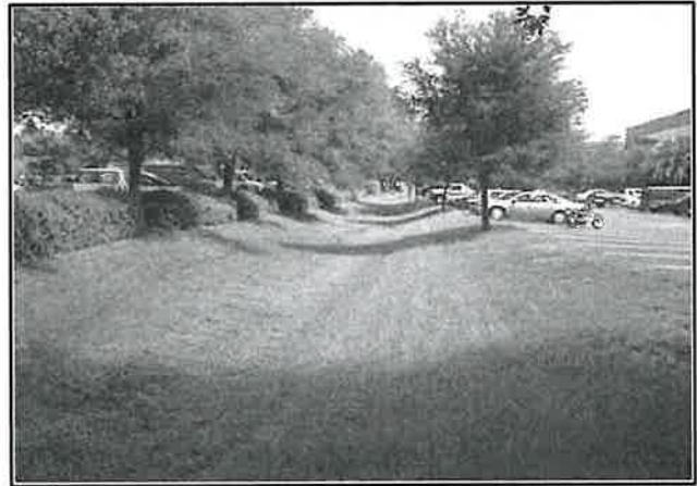
Figure 20. Vegetated swale (Virginia DCR 2011).
