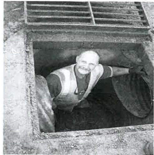
Figure 189. Cleaning a sediment trap.
