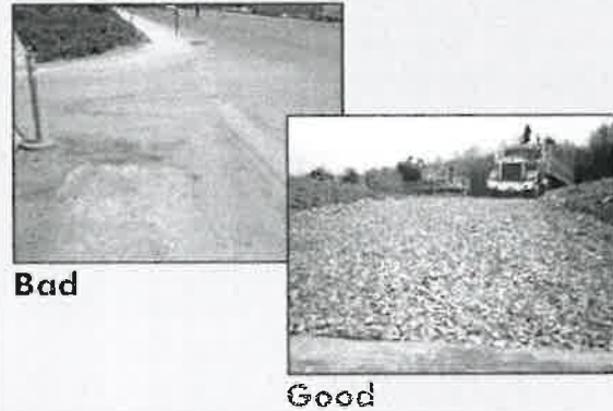
Figure 102. Stabilized gravel construction entrance examples (EPA 2003).
