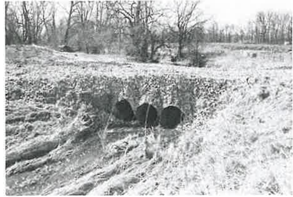
Figure 149. Temporary stream crossing using culverts (Ohio EPA 2014).
