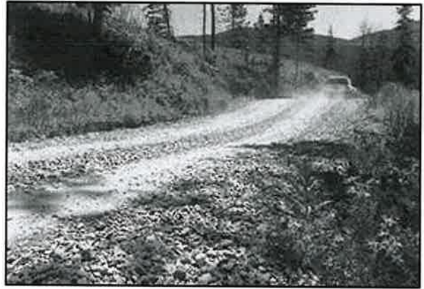
Figure 198. Remote access road with rolling drain dip (University of Idaho 2015).
