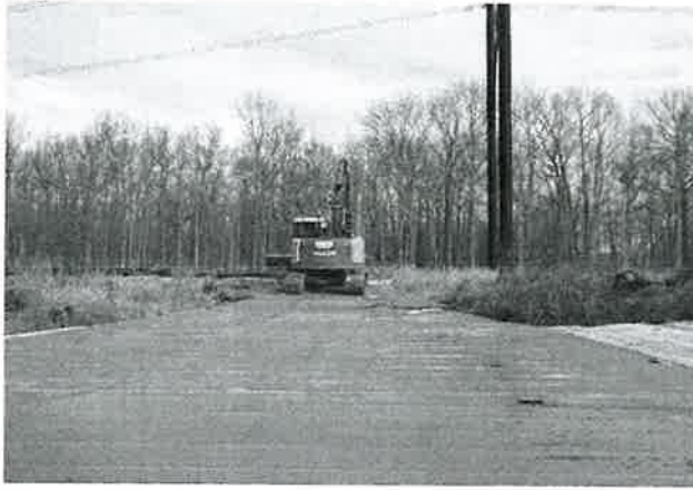
Figure 104. Construction mat ( Matrax ).
