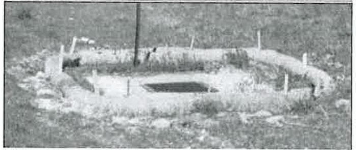
Figure 182. Inlet protection wattle (ITD 2014).
