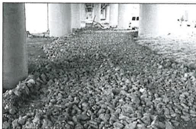
Figure 108. Temporary construction access road (ITD 2014).
