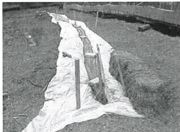
Figure 176. Floc logs located in channel (Applied Polymer Systems).
