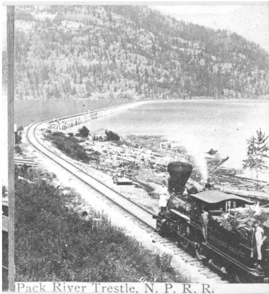
Figure 5. "Northern Pacific balloon stack steam engine approaching the Pack River Trestle across to Trestle Creek, circle late 1800s." Used with the permission of the BCHS and consistent with the fair use doctrine of the US Copy Right (cf 37CFR201.2 (a) (3)).
