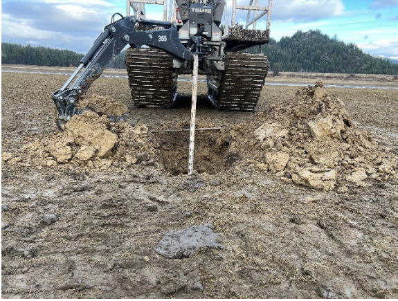
Figure 14. Excavation of GT004.
