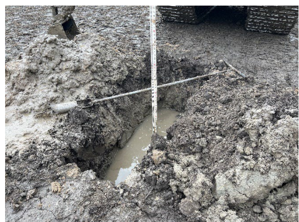
Figure 18. Excavation of GT013, water fill.
