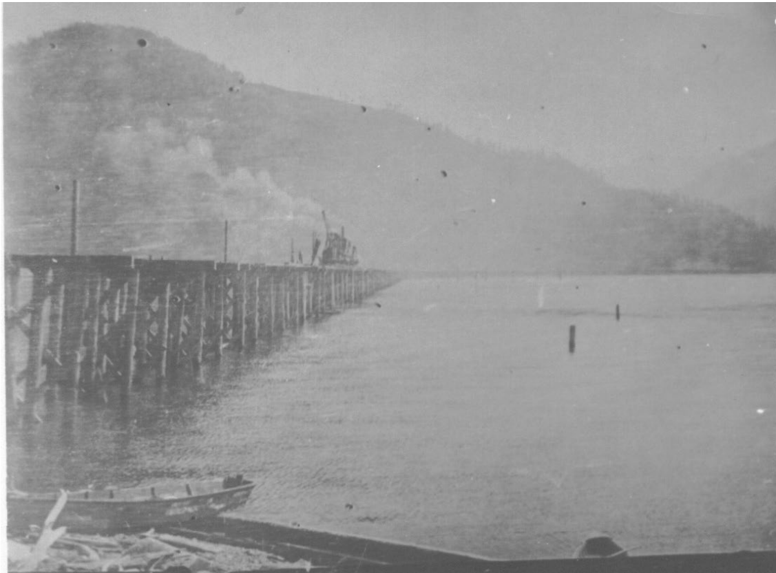
Figure 4. "Photo of Northern Pacific Railroad trestle across the Pack River under construction, 1882." Used with the permission of the BCHS and consistent with the fair use doctrine of the US Copy Right (cf 37CFR201.2 (a) (3))
