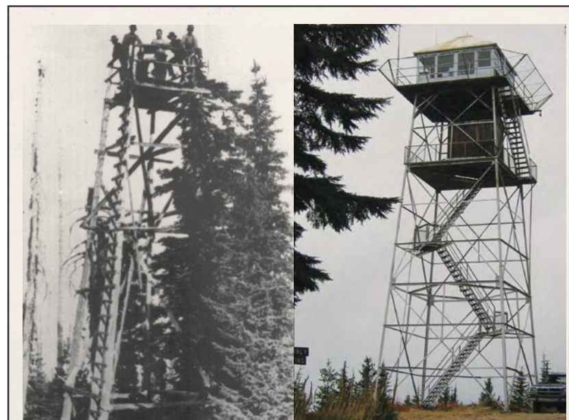
The Bertha Hill Lookout stands 29 miles north and east of Orofino. It has been manned by CPTPA every year since 1900. The first “tower” was a 15 foot hemlock snag. The current lookout is a 50 foot steel tower.
