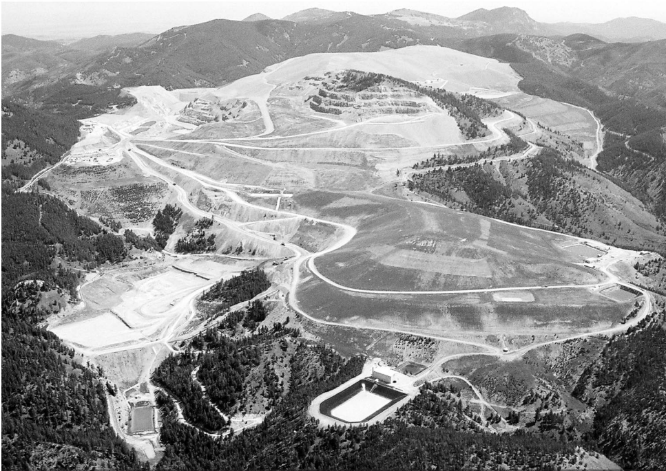
Landusky 2004 Reclamation near completion
